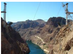
The O'Callaghan/Tillman memorial bridge under construction
