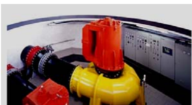
Small Run-of-River Hydroelectric Turbine
