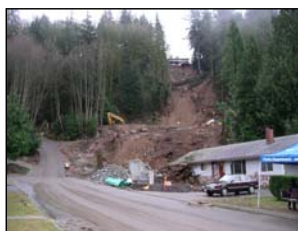
The aftermath, Riverside Drive
